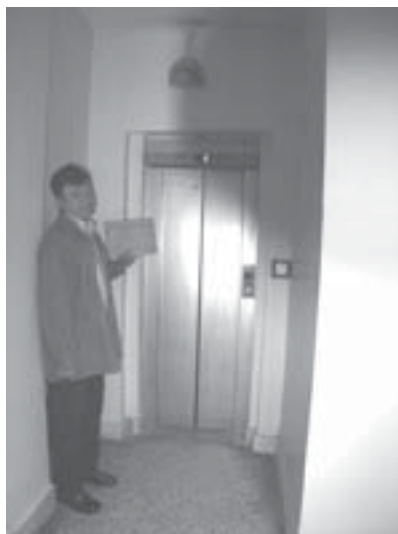
Inaccessible lift in the economic faculty in Sarajevo, BiH
