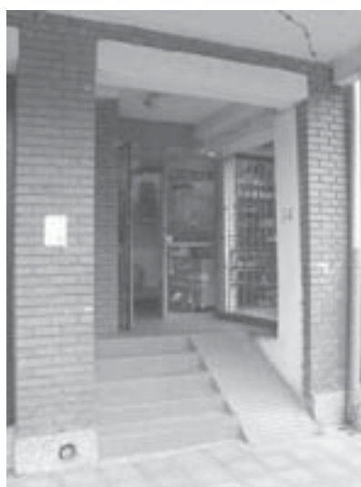
Apartment building in Skopje, Macedonia
