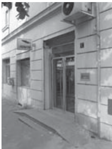
Accessible entrance to post office in Belgrade, Serbia
