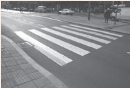
New street in Belgrade, kerbs are not cut on both sides of the street
