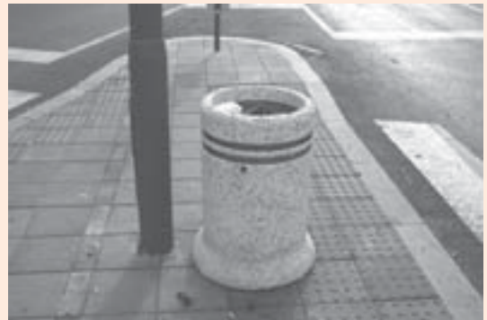
Trash bin obstructs textured pathway
